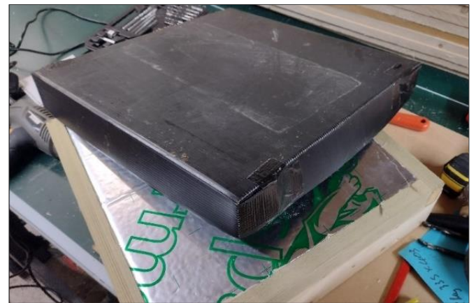
A piece of 4mm Correx cut and taped makes a cheap and effective cover (roof) for this insulation frame.
